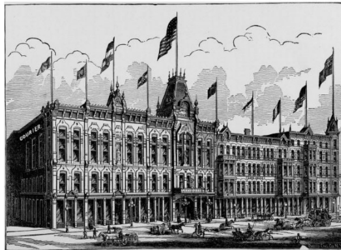
SCHULTZ'S OPERA HOUSE, Zanesville, Ohio.
